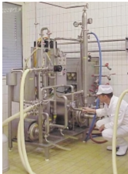
Picture 1: The milk was concentrated in this microfiltration plant
