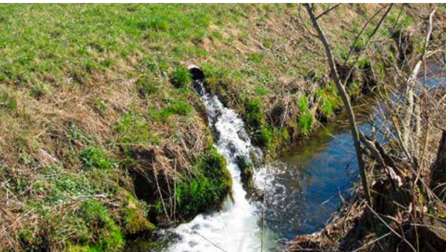
Drainage pipe discharging into a watercourse. (Photo: Volker Prasuhn, Agroscope)
