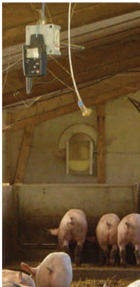
Figure 12. Sensors must be installed beyond the reach of animals.
