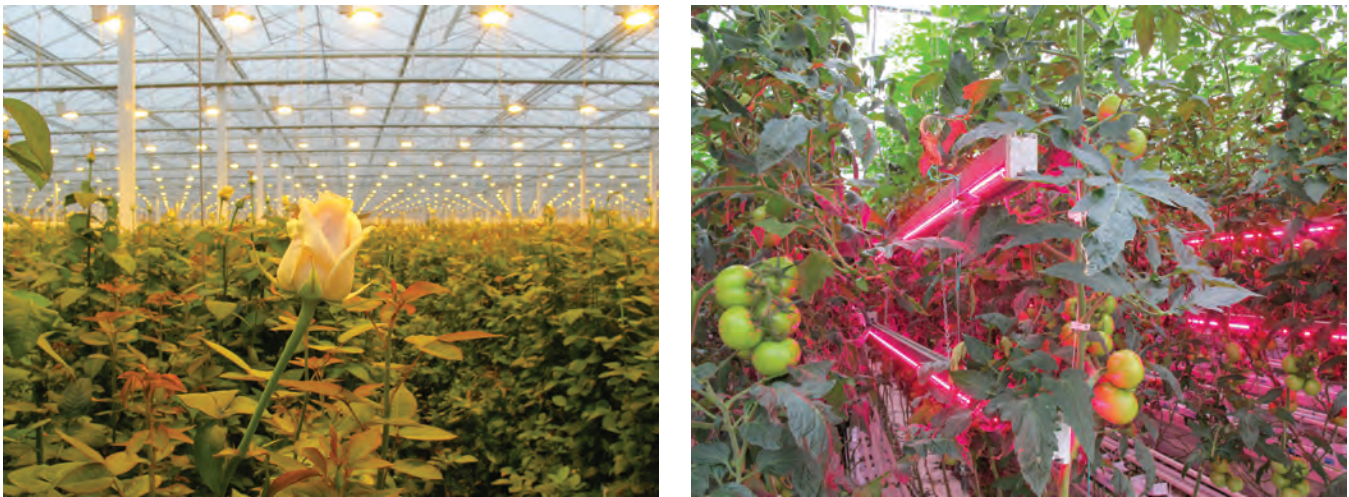
Figure 6. High-pressure sodium fixtures mounted over a rose crop (left) and LED fixtures with a magenta color mounted within a tomato crop (right) (photos by A. J. Both).
