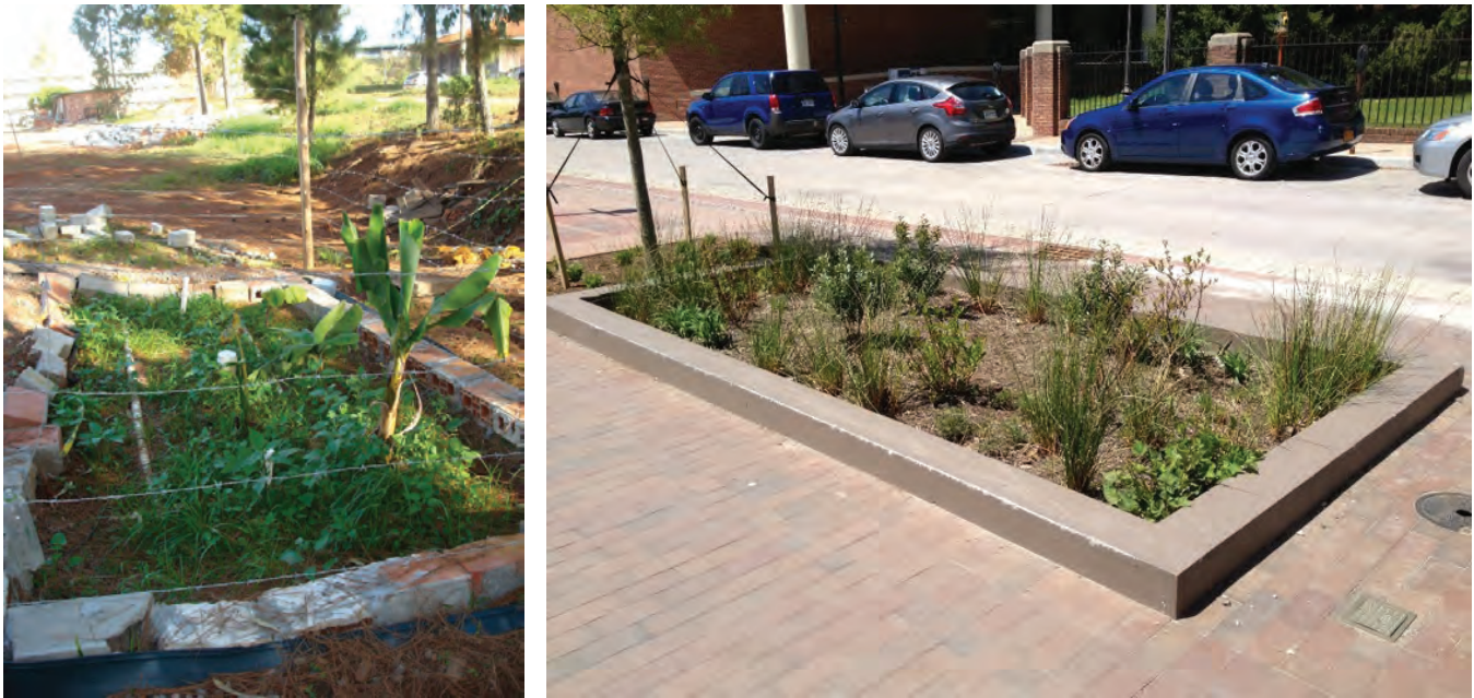
Figure 2. Bioretention cells for urban stormwater control in Brazil (left) and the USA (right). These cells are designed to temporarily store water, allowing sediments to settle, and using plants for nutrient uptake. Note the use of local native vegetation.
