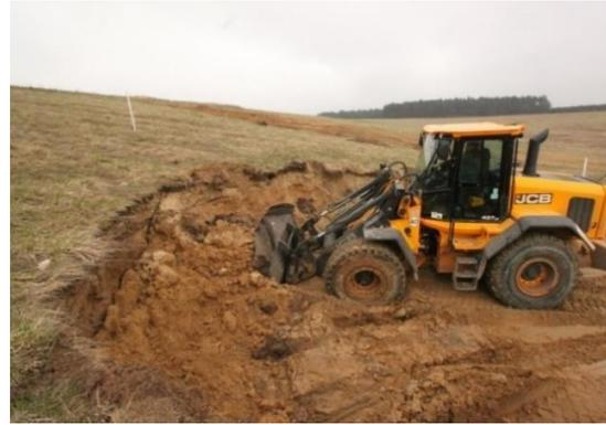
**Figure 14: Creation of break-off edges**
