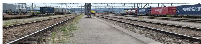
Fig 4: On the left: rail track A4, 1 month after glyphosate treatment, on the right: rail track A4 after the 2nd hot water treatment (30.06.2020).
