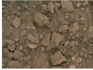
Aggregates partly washed out, surface nevertheless rough/uneven
