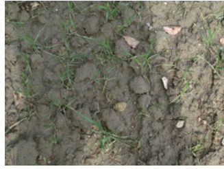
Aggregates washed out, surface silty, kneaded, few permeable
