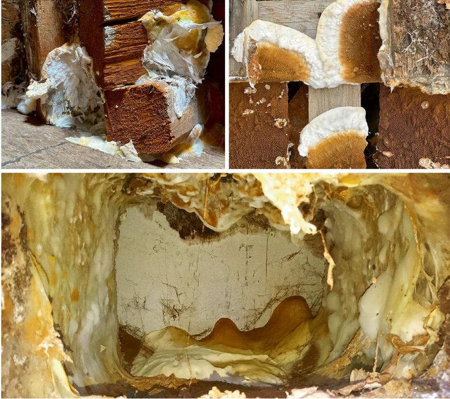
**Fig. 3.21** Different stages of development of dry rot (*Serpula lacrimans* (Wulfen) J. Schröt.) on construction timber. The mycelium, white or creamy yellow initially, becomes brownish yellow to rust-coloured as the fungus develops. (Photographs © Paraxyl Sàrl, Switzerland)
