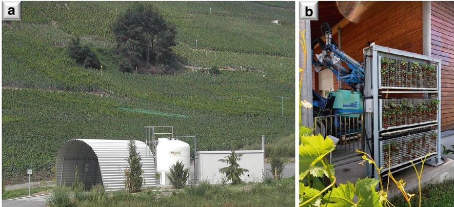
**Fig. 8.44** Collective sprayer cleaning and recycling areas in or next to vineyards allow the recovery of residues, waste and contaminated cleaning water (a), which can then be properly recycled in biologically active systems (b)
