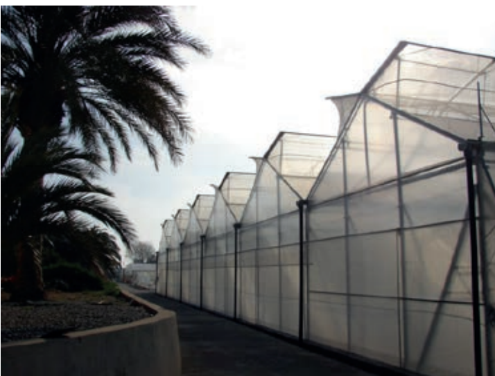
Newly designed greenhouses with improved ventilation. Fundación Cajamar, Almería (Spain).
