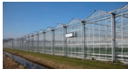
Dehumidification units in organic tomato greenhouse in the Netherlands.
