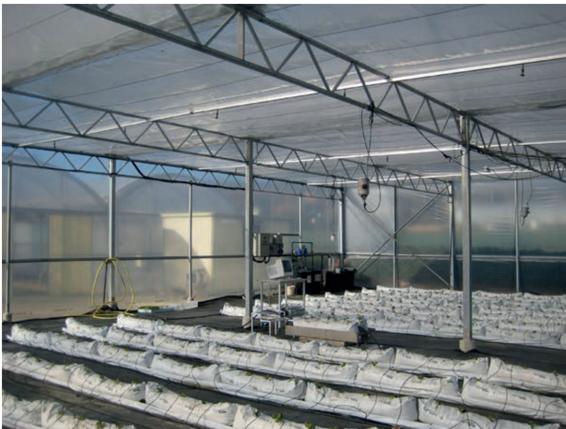
Thermal PE screen in a high tech Southern European Greenhouse
