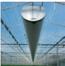
Dehumidification units in organic tomato greenhouse in the Netherlands.
