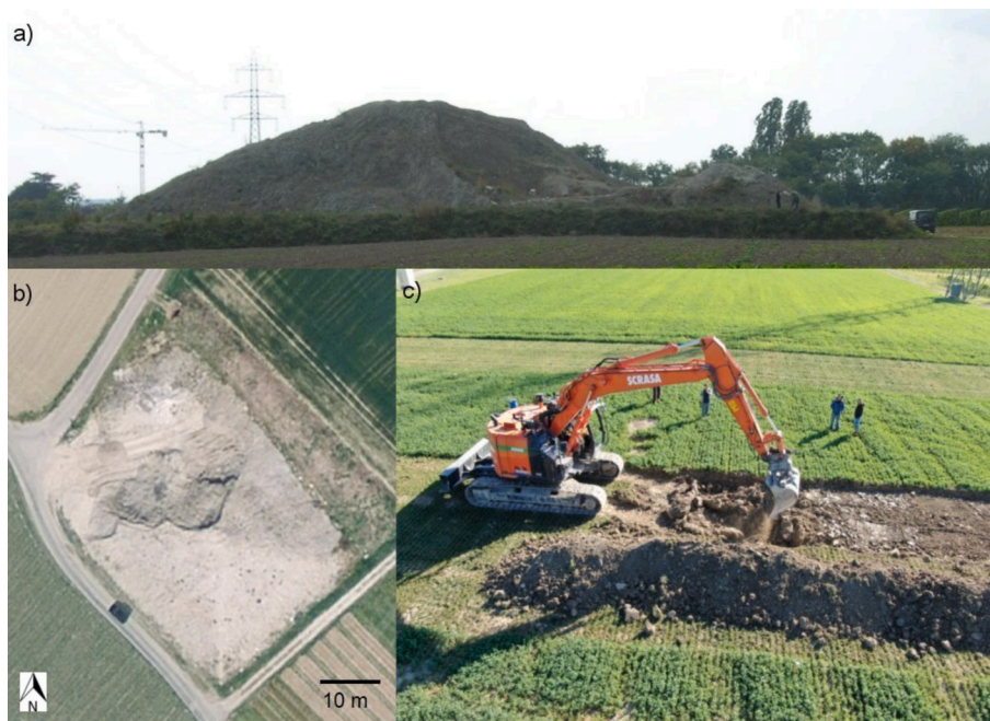
Fig. 1. (a) The pile of excavation material seen from the side. Note the van and the two persons at the right of the image for scale; (b) the pile of excavation material seen from above in spring 2015; (c) mechanical subsoil loosening with a digger in June 2020.
